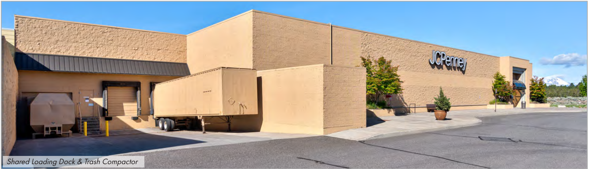
Anchor Building G from West Parking Lot
